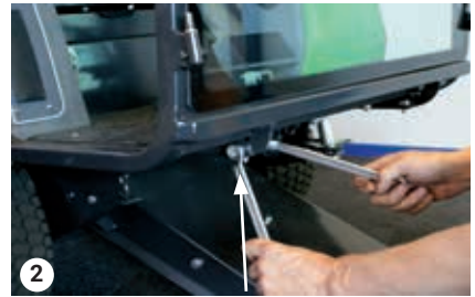
Bolts under base plate
