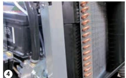
Clean coolers using compressed air
