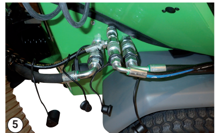
Hydraulic hoses attached – front
