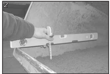
Measure horizontal in, vertical down
