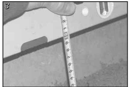
There should be 10 cm down to the sand
