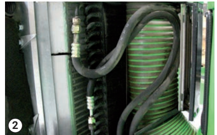
Wash the radiators with clean water
