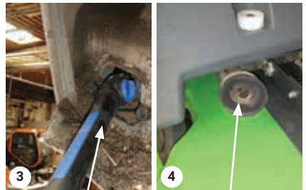
Clean filter inside and out and Clean pipe system at waste tank with high pressure unit
