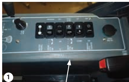
Panel de control
